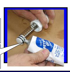
Installing Plunger assembly C6513P into faucet body
